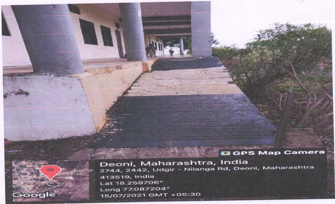
Ramp for Disabled Students
