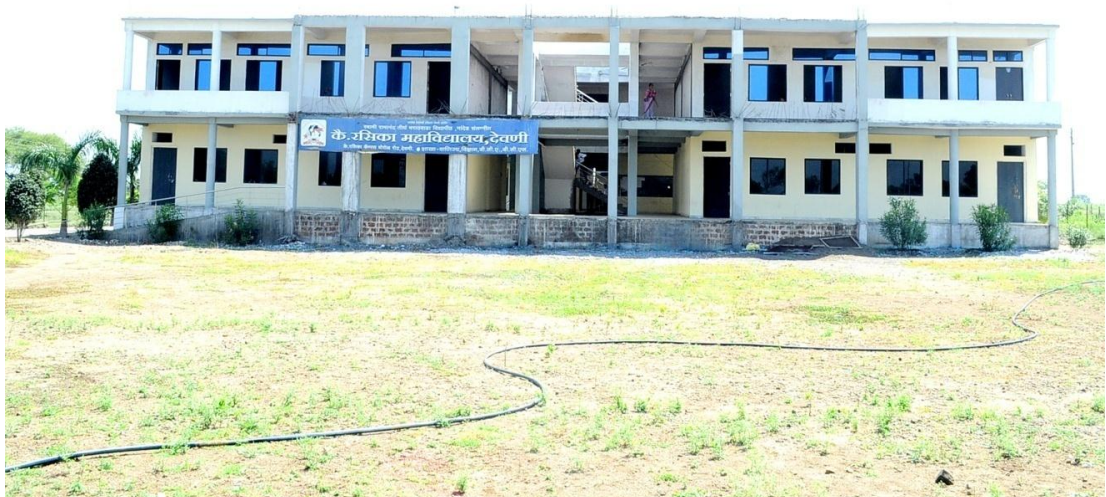
Figure 4.2 College building (Side View).
